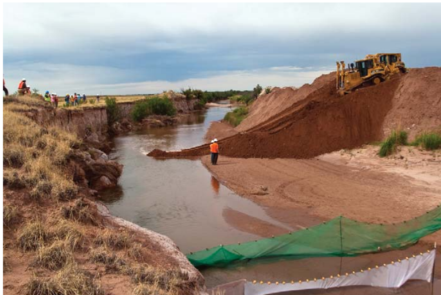
Figure 1. Pecos River Restoration Project-reopening a historic meander and closing a channelized reach (2009) © Ken Stinnett
