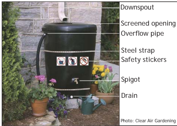
Figure 13. Components of a passive rainwater harvesting system
