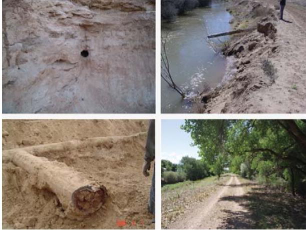
Figure 3. Current Albuquerque levee conditions
