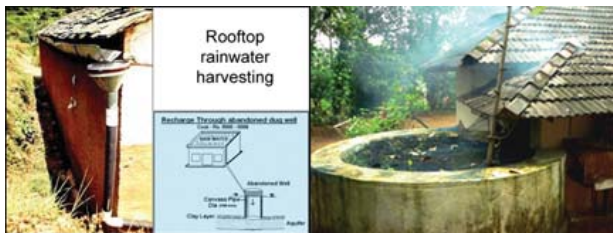
Figure 17. Artificial recharge with roof water is mandated in some provinces in India
