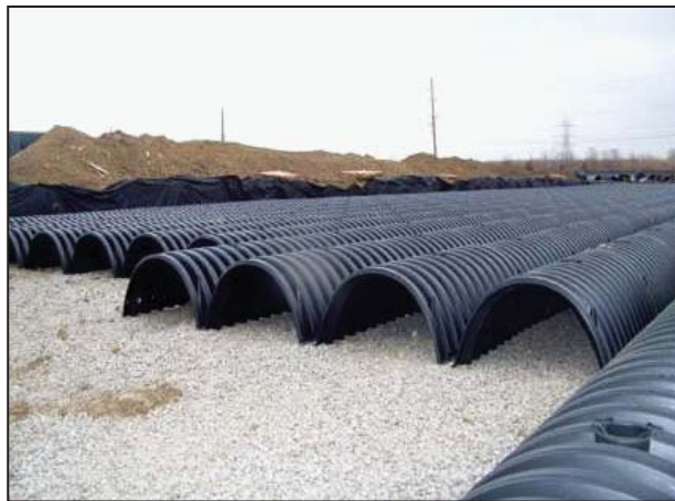
Figure 20. Wrapped corrugated metal pipe that has been filled with gravel
