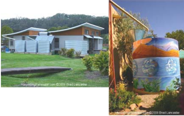
Figure 9. Lot scale rainwater harvesting
